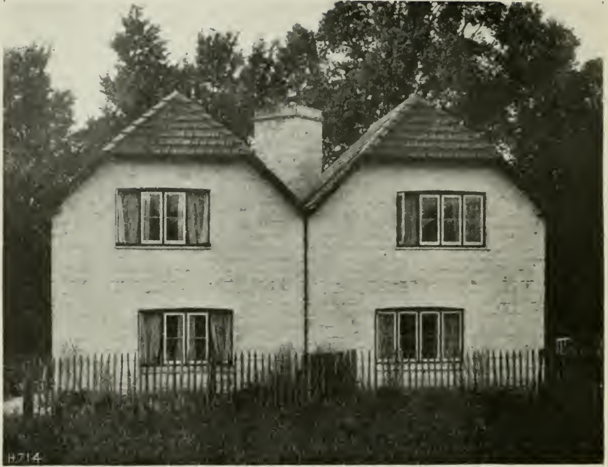
FIG. 25.—MR. ST. LOE STRACHEY'S COTTAGES BUILT OF CONCRETE BLOCKS.
